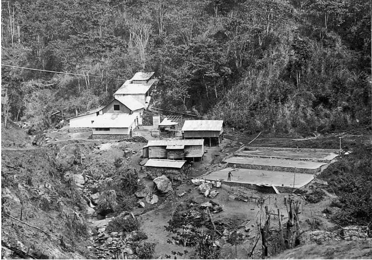
Figure 7. Hacienda Cincinnati mill complex. It housed the electric generator, coffee bean processing machinery, and workshops. The coffee bean drying pads can be seen on the right. I remember visiting it as a child in awe of the giant wheels and conveyer belts still in operation.
